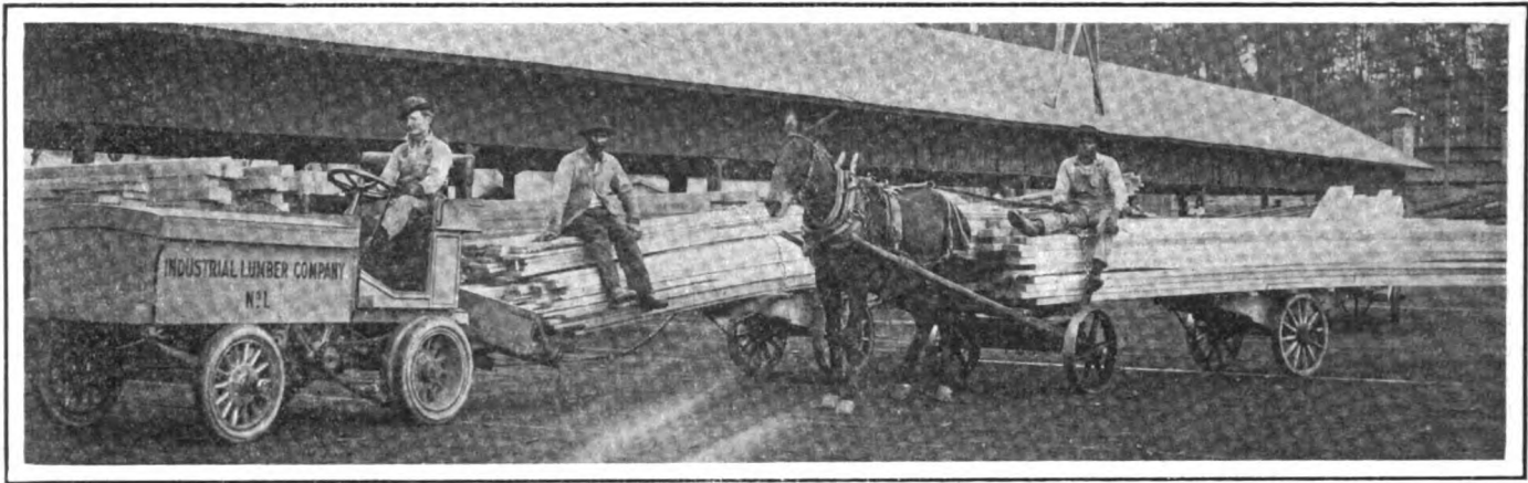
Two-ton electric lumber tractor with traller. The batteries are situated in a single front compartment and the lumber is mounted on a two-wheeled truck. The old and new methods are contrasted
